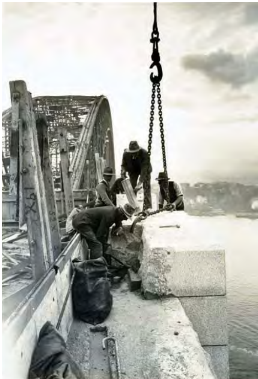
Left, stonemasons completing the south-east pylon of the Harbour Bridge. This photograph was taken on 2 September 1931 by D. J. Fraser. (SLNSW, Government Printing Office, PXA 624, vol 2). Below, the Bridge in 1932 by Samuel Wood. The south-east pylon is in the foreground. (SLNSW ON275/59)
